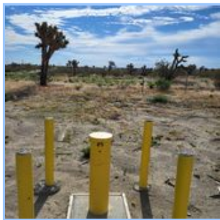
Oeste Recharge Facility
