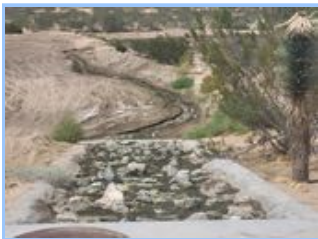
Pipes Wash Recharge
