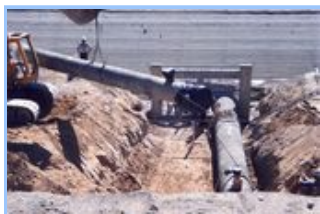
White Rd TO Construction.jpg
