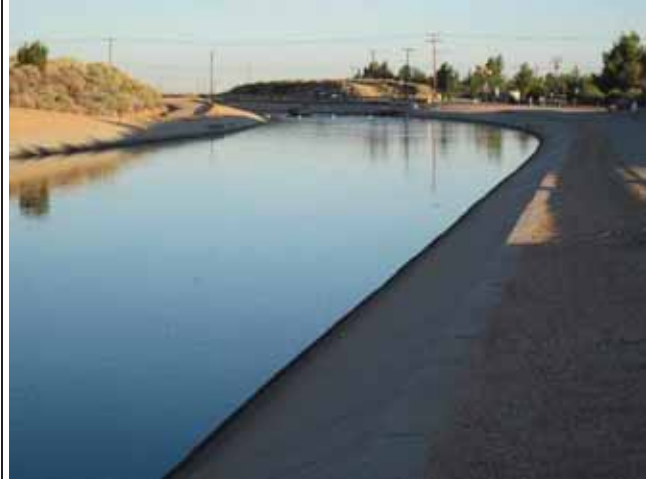
08/28/12, Camera A2, Frame 1076: View towards Rancho Road
