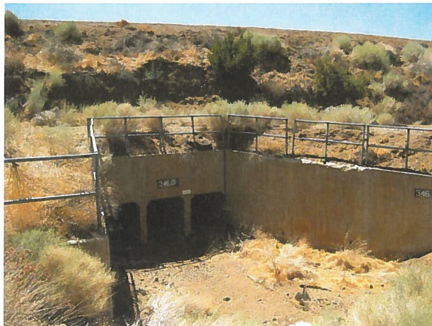
Figure 6. Triple Box Culvert, facing south
