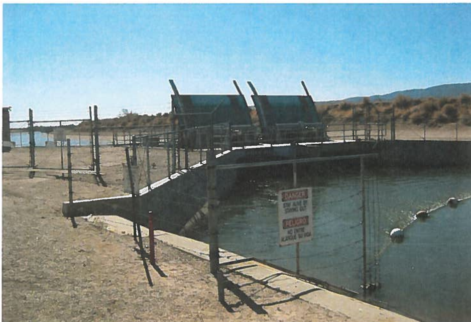
Figure 2. Canal Check Structure, facing southwest
