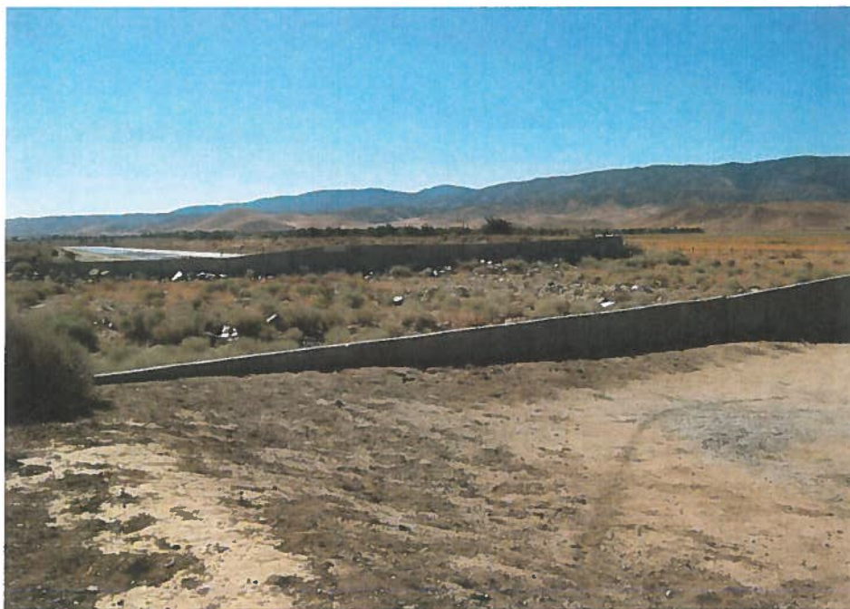
Figure 2. Box Siphon, facing southwest
