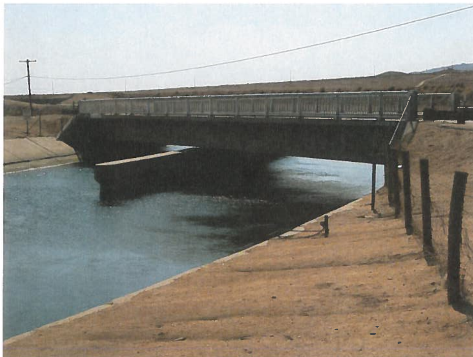
Lancaster Bridge and EBA Canal, facing northwest
