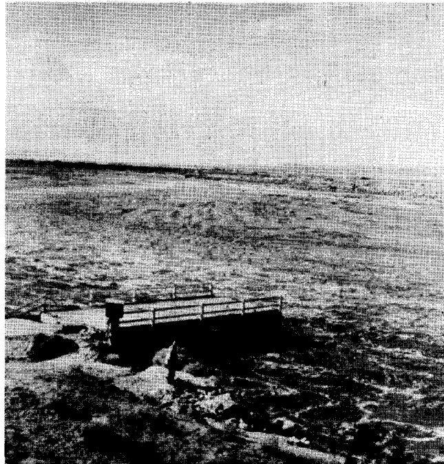
Figure 17.--Indian Trail Road bridge between Helendale and Hodge. Picture shows approach to the bridge washed out. February 1969
