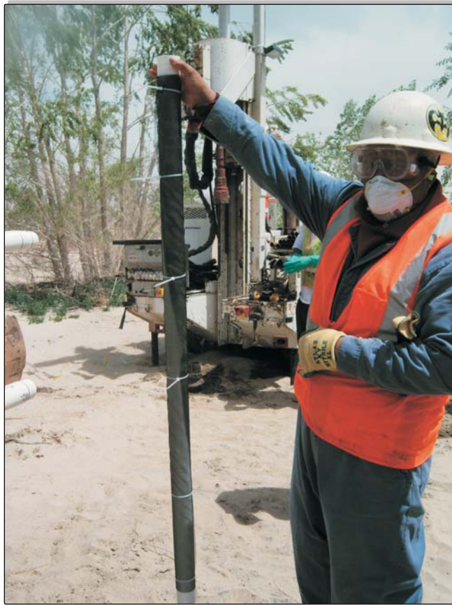
Well screen installation
